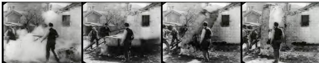
Figure 9 Demolition of a Wall by the Lumière brothers shows the action in reverse too
